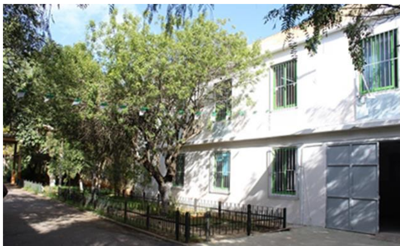
The building studied
